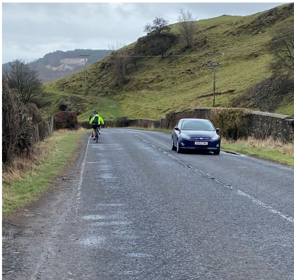
Figure 2 - Current provision at NCR7 entrance
