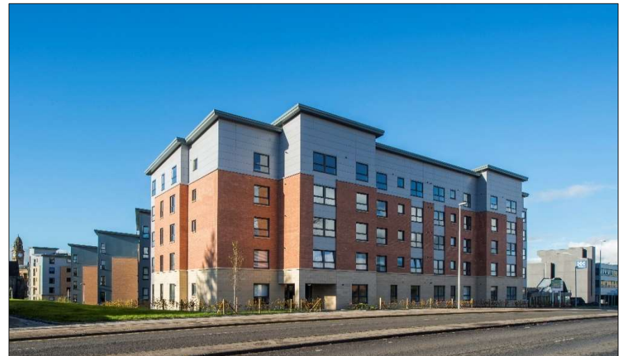
Mixed Tenure Purpose built development for older people, Paisley Town Centre (Link Group)
