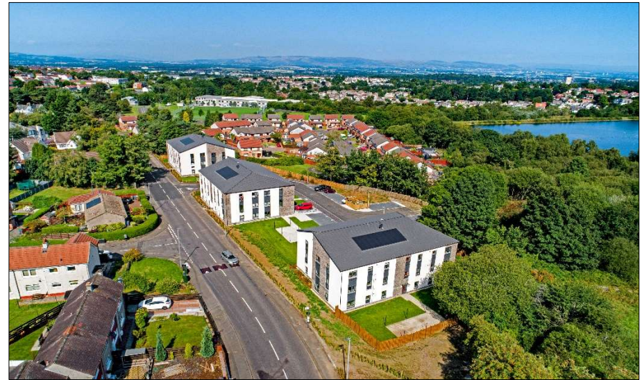
Link Group development, Amochrie Road, Paisley, Contractor JR Group
