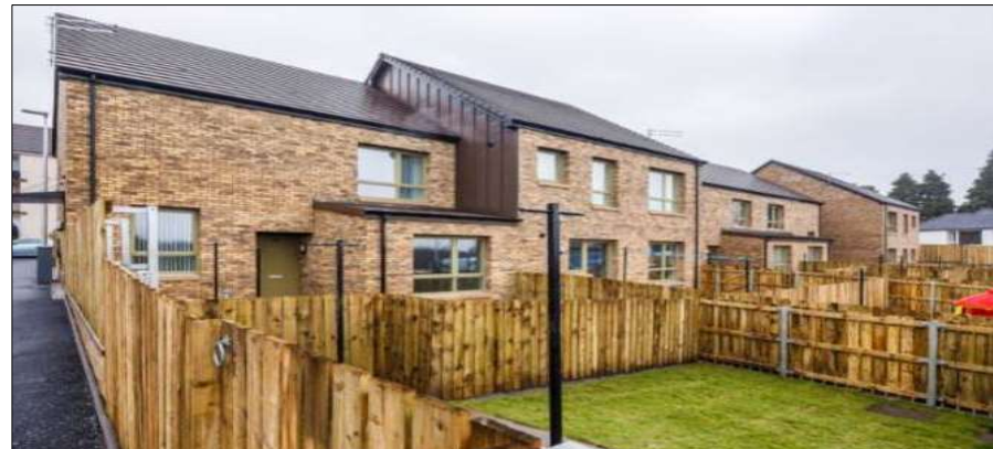
Williamsburgh Housing Association development, Milliken Road, Kilbarchan
