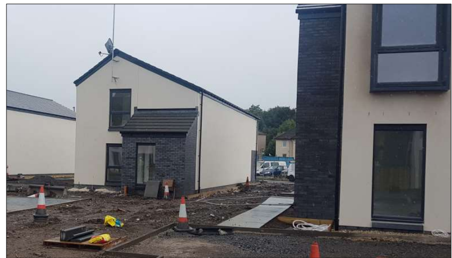
Link Group development under construction, Thrushcraigs, Paisley
