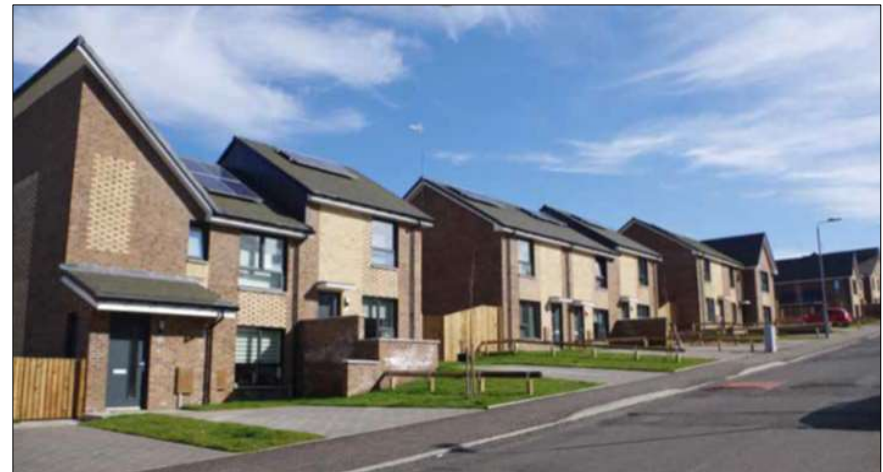
Renfrewshire Council new build development, Johnstone Castle
