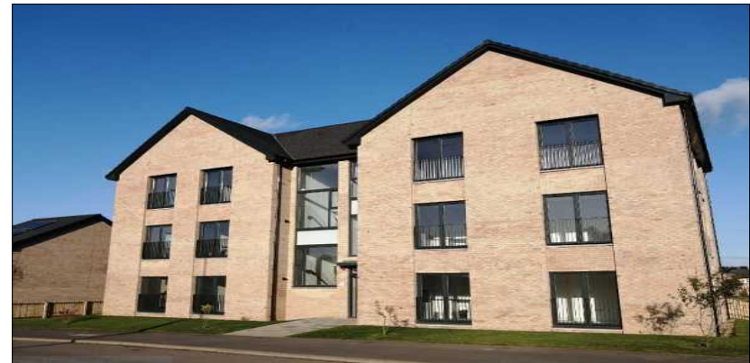
New Build Council Homes, Dargavel Village, Bishopton (Amenity and General needs flats)
