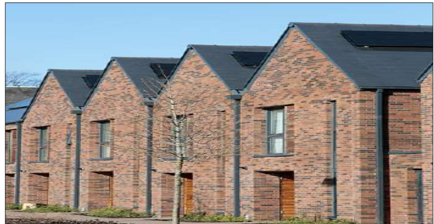
Development with Solar PV to reduce energy costs for tenants, Paisley
