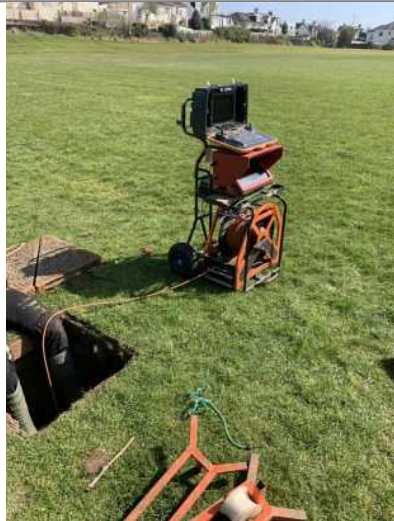
Manhole / Access Point: MH1 Location
