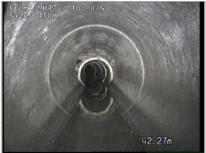
Junction at 10 o'clock, diameter 150mm
