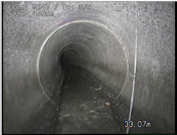
Junction at 2 o'clock, diameter 150mm
