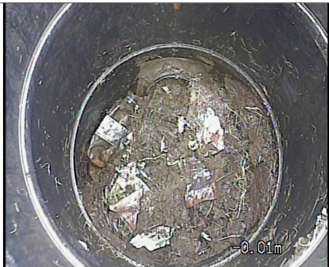
Manhole / Access Point: POINT A MH Internal
