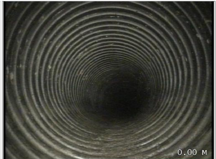
Water level 5% height/diameter
