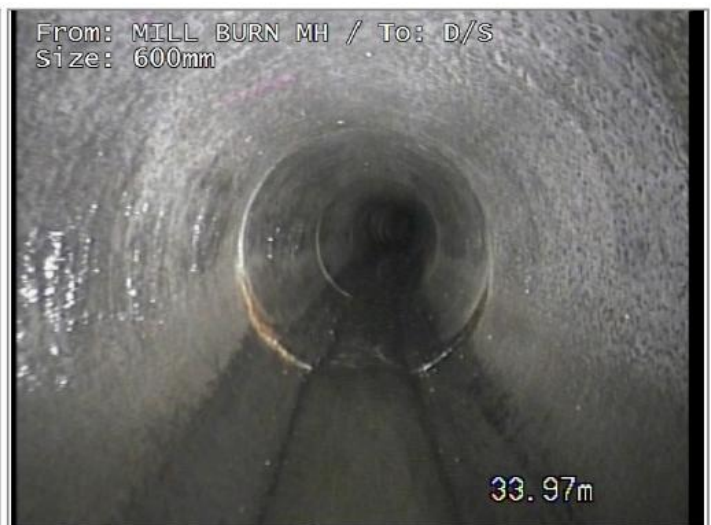
Junction at 2 o'clock, diameter 150mm
