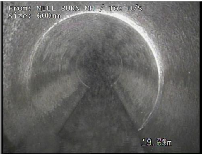
Junction at 9 o'clock, diameter 150mm
