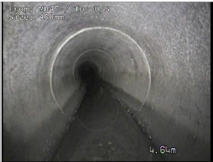
Junction at 10 o'clock, diameter 150mm
