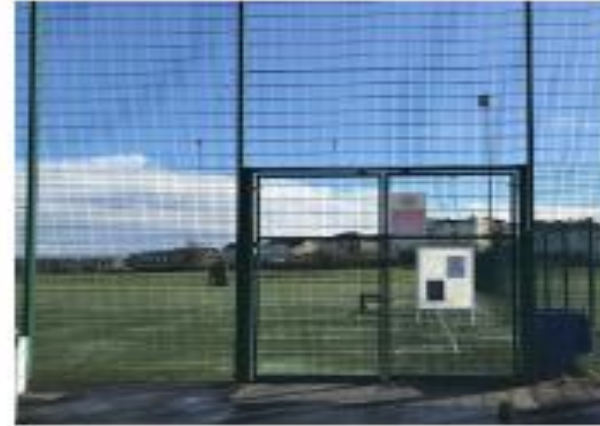
EXISTING GATE 1 (3.18m HIGH x 2.95m WIDE)
