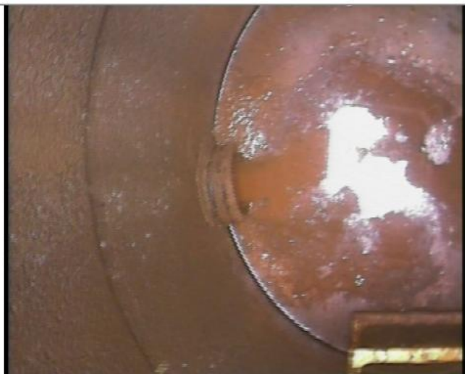
POINT C MH Internal
