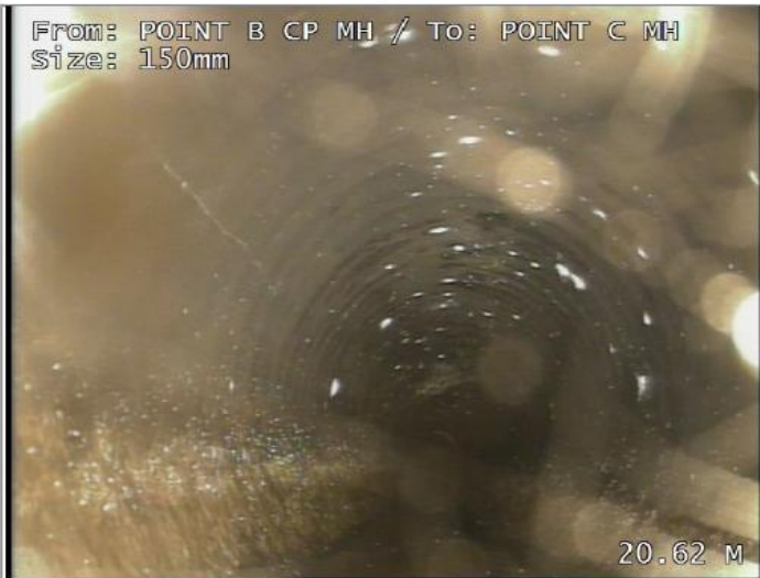
Water level 10% height/diameter, Finished
