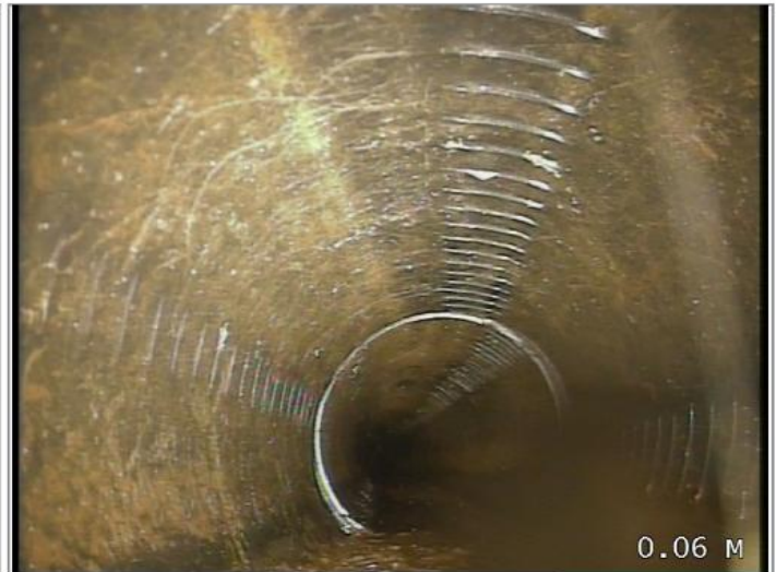
Water level 5% height/diameter
