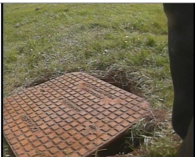
Manhole / Access Point: POINT B CP MH Location
