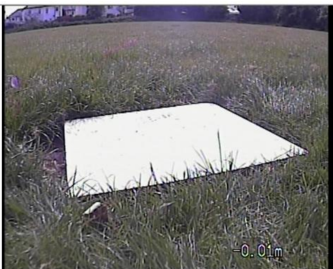
POINT A MH Location
