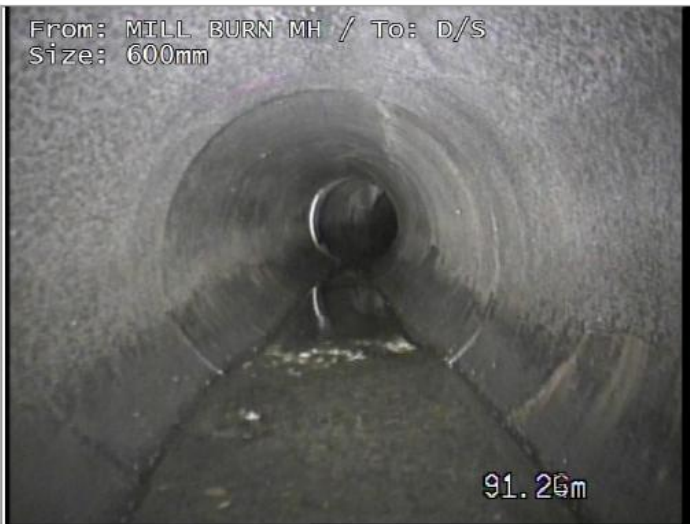
Junction at 2 o'clock, diameter 150mm
