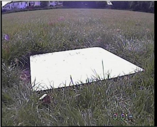
POINT A MH Location
