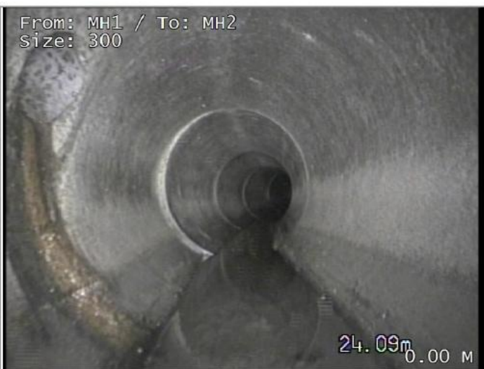
Junction at 10 o'clock, diameter 100mm
