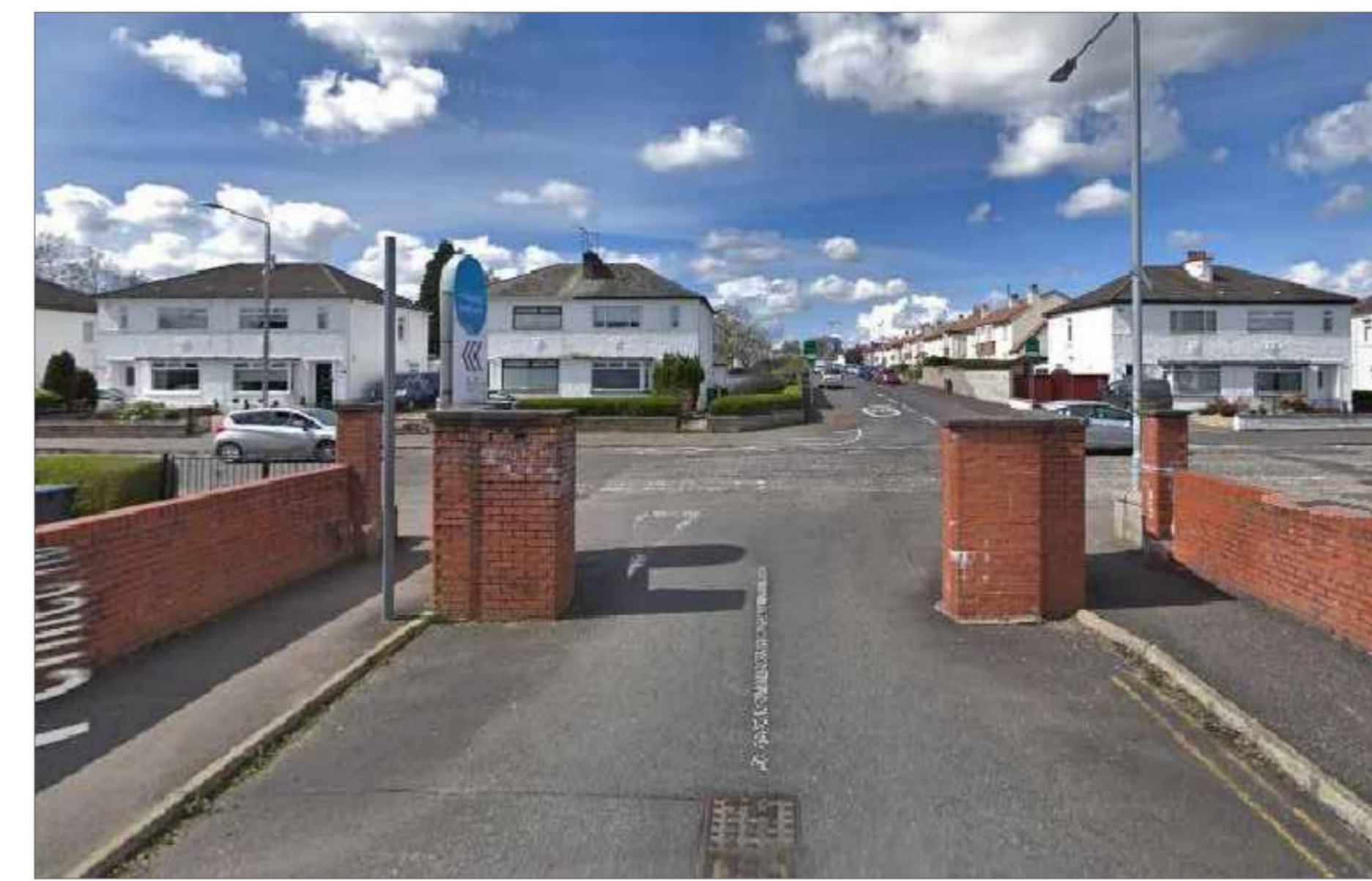
EXISTING ENTRANCE (PHOTO 2018) NOTE AVAILABLE WIDTH BETWEEN PIERS APPROX. 3831mm DOES NOT ALLOW FOR 2 CARS TO PASS MINIMUM ACCESS WIDTH REQUIRED FOR 2 CARS TO PASS = 4700mm (REFER TO SCOTTISH NATIONAL ROADS GUIDE SECTION 3.1.3 DESIGN DETAILS)
