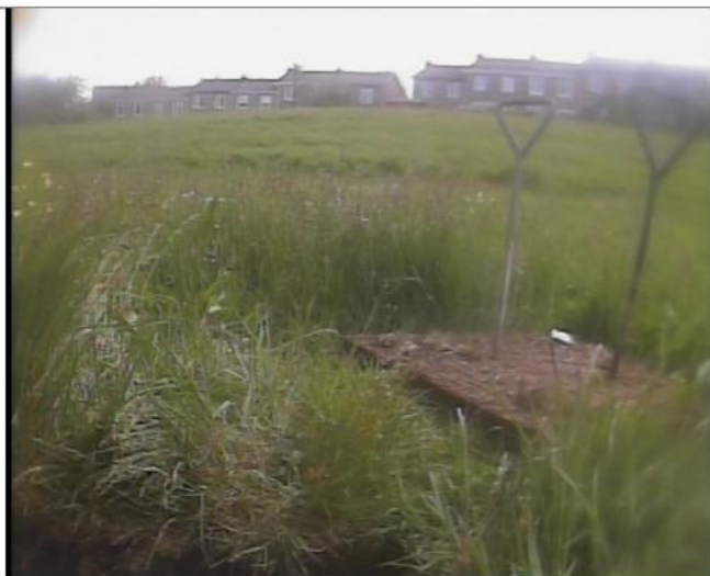
Manhole / Access Point: POINT D STORAGE TANK Location
