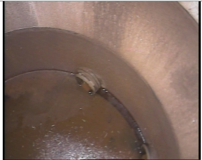
POINT D STORAGE TANK Internal
