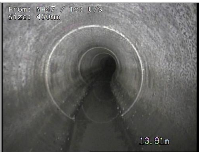
Junction at 2 o'clock, diameter 150mm
