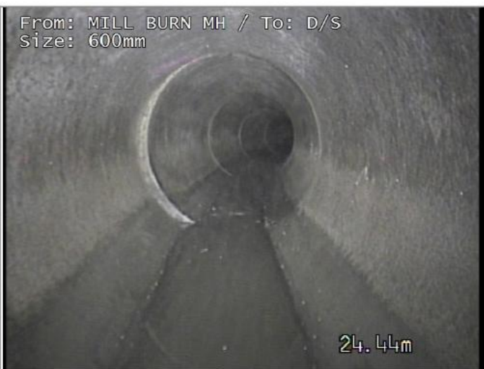
Junction at 10 o'clock, diameter 150mm
