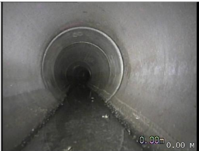
Start node type, manhole, reference MH1
