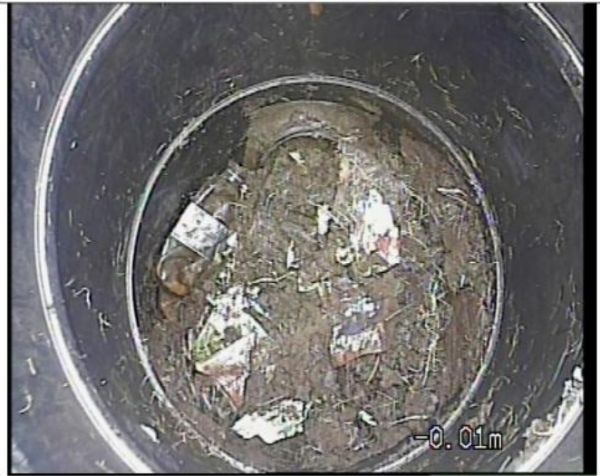
POINT A MH Internal
