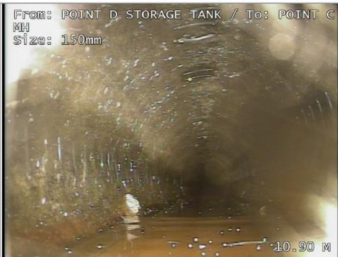
Water level 10% height/diameter, Start
