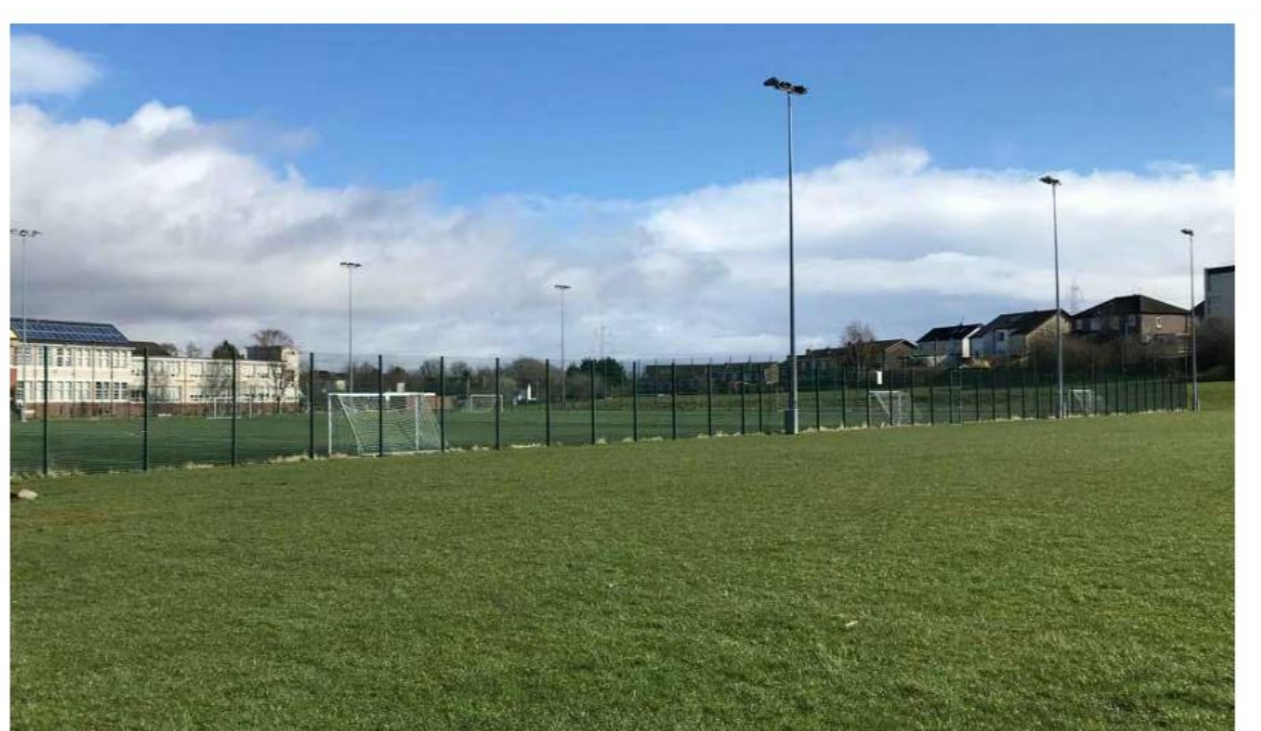
EXISTING ABACUS 15m HIGH LIGHTING COLUMNS
