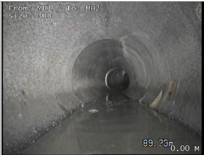
Junction at 2 o'clock, diameter 100mm
