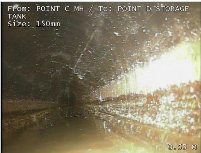
Water level 25% height/diameter, Start
