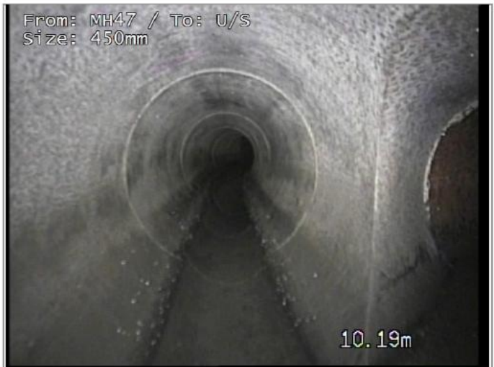
Junction at 3 o'clock, diameter 450mm
