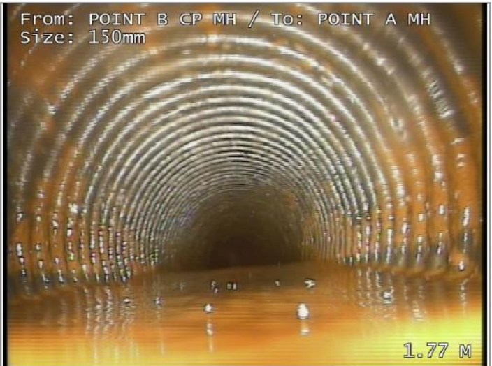
Water level 50% height/diameter, Start
