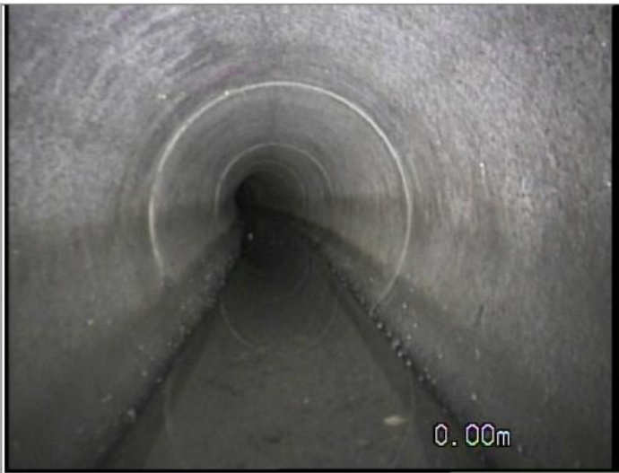
Start node type, manhole, reference MH47
