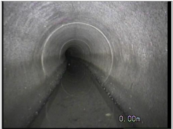
Water level 5% height/diameter
