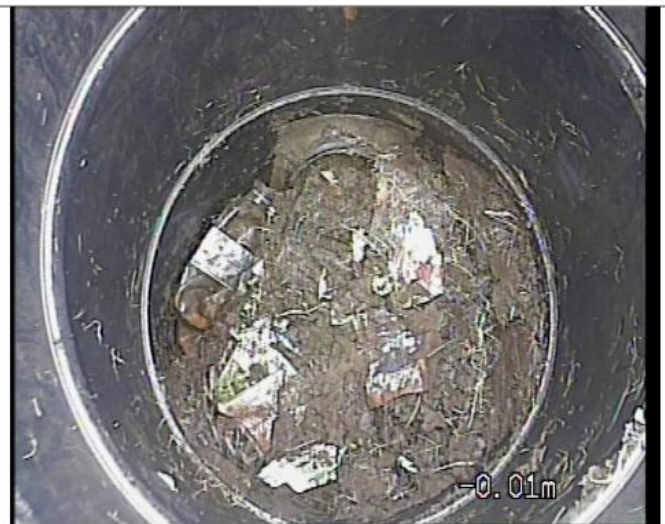
POINT A MH Internal
