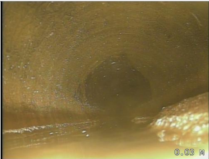
Start node type, manhole, reference POINT C MH
