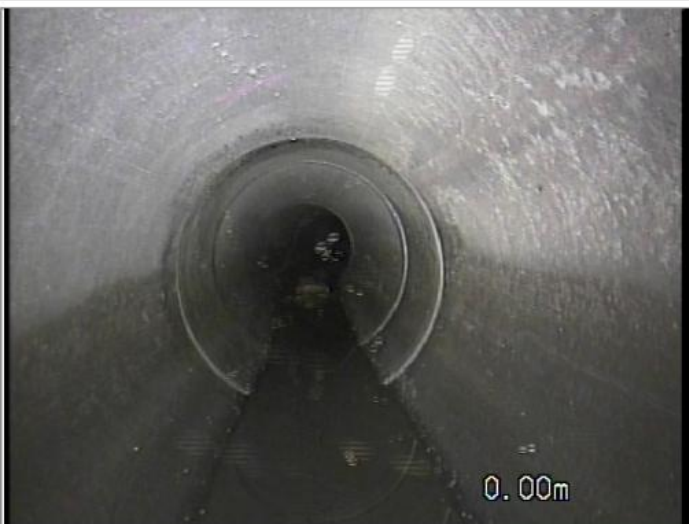
Water level 5% height/diameter
