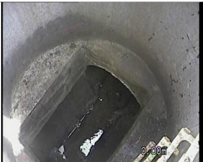
Manhole / Access Point: MILL BURN MH Internal
