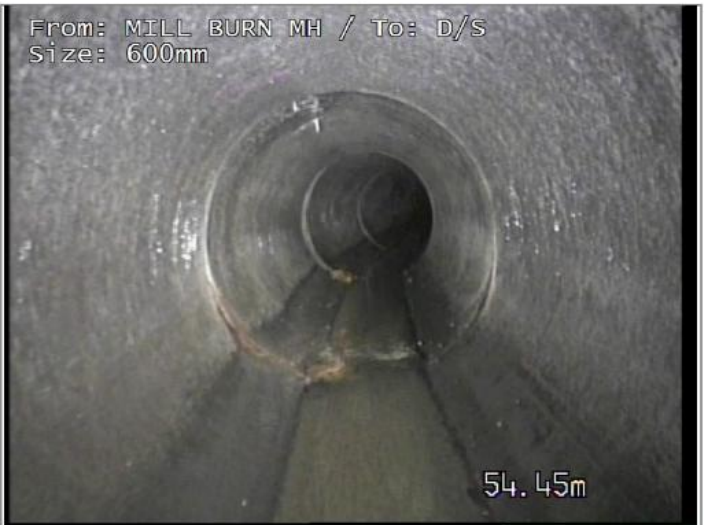
Junction at 2 o'clock, diameter 150mm
