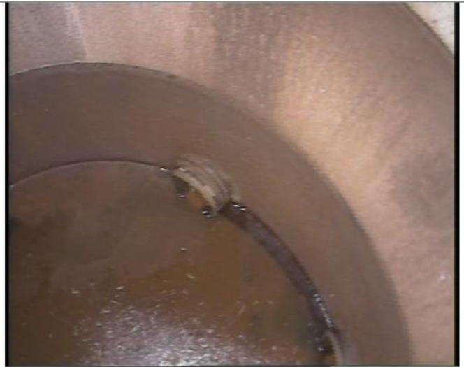
POINT D STORAGE TANK Internal
