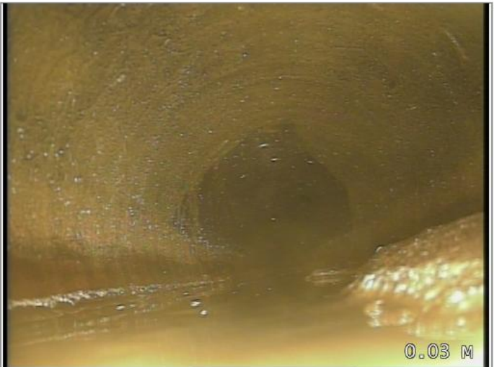
Water level 5% height/diameter
