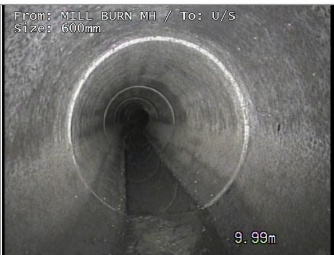
Junction at 2 o'clock, diameter 150mm
