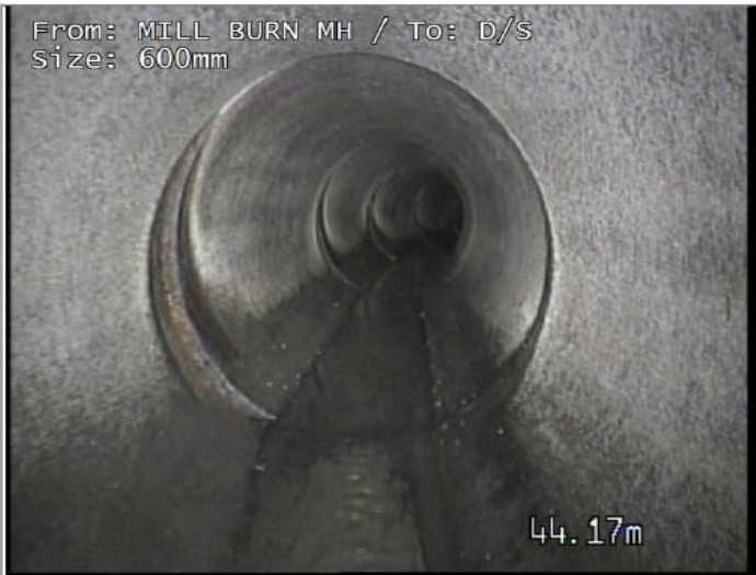
Junction at 11 o'clock, diameter 150mm
