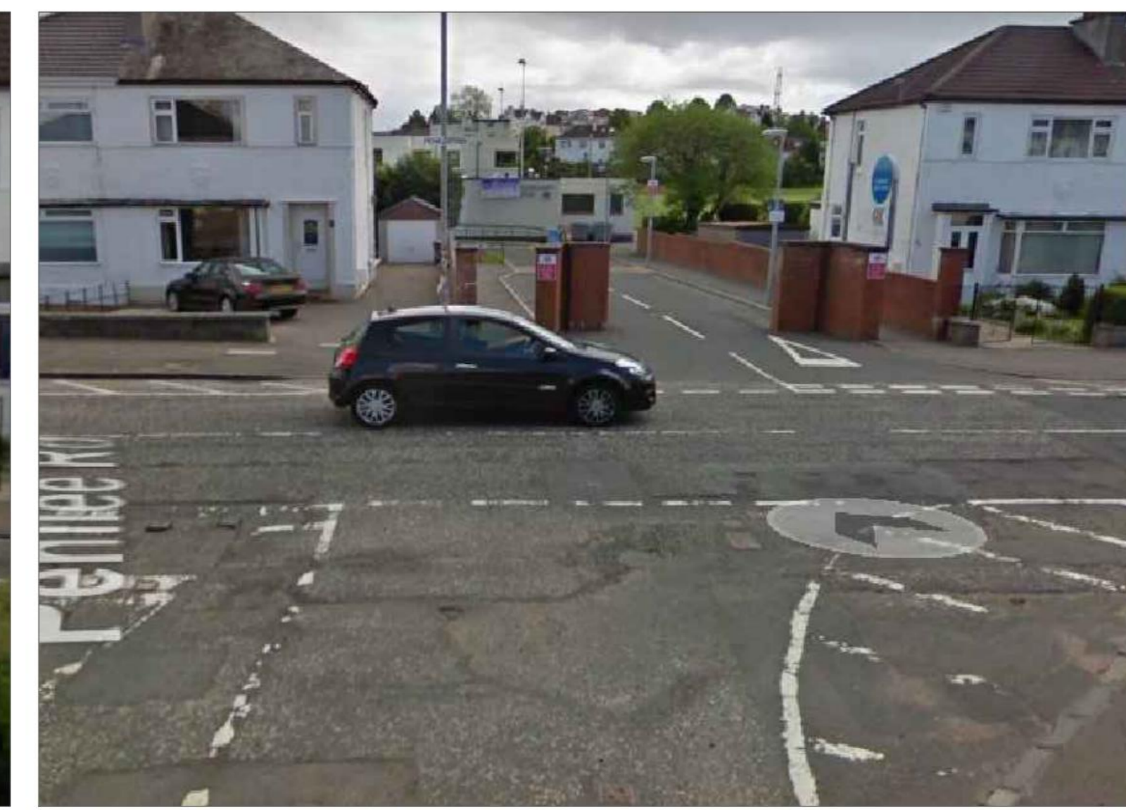
EXISTING ENTRANCE (PHOTO 2011) REFURBISHMENT & NEW EXTENSION COMPLETED NOTE NEW FOOTPATHS, UPSTAND KERBS & SPEED CALMING MEASURES UPON ENTRY INTO THE ACCESS ROAD TO THE SITE
