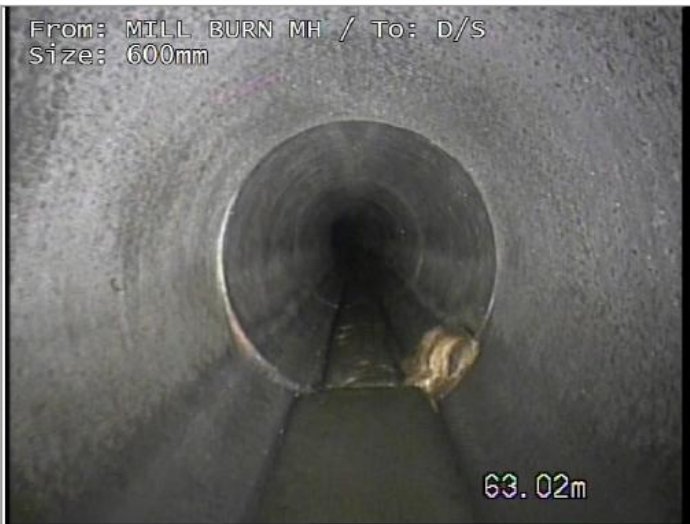
Junction at 10 o'clock, diameter 150mm
