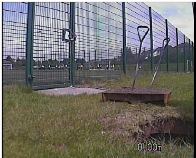
Manhole / Access Point: MILL BURN MH Location
