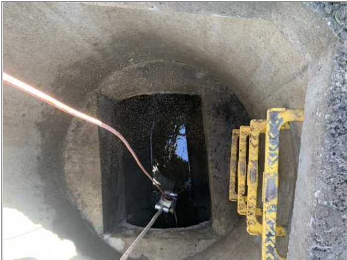
Manhole / Access Point: MH1 Internal
