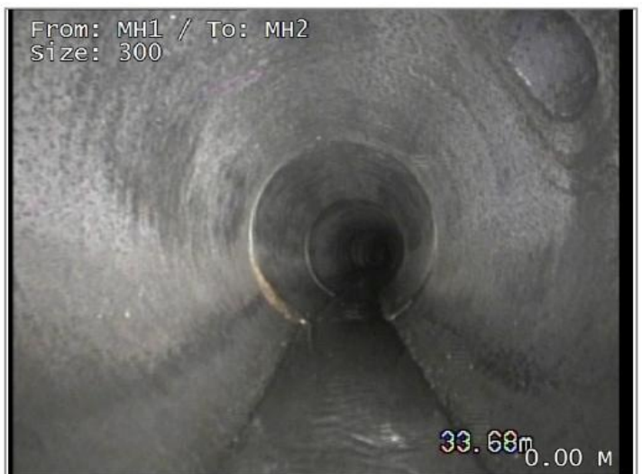
Junction at 2 o'clock, diameter 100mm
