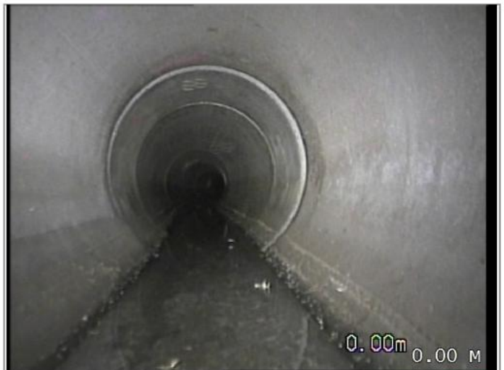
Water level 5% height/diameter
