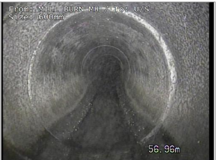
Junction at 10 o'clock, diameter 150mm
