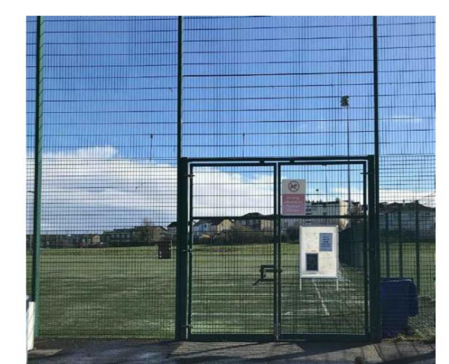
EXISTING GATE 1 (3.18m HIGH x 2.95m WIDE)
