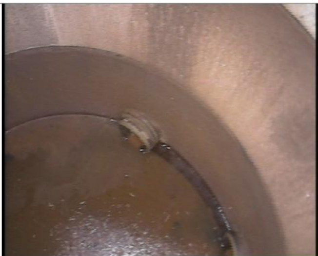
Manhole / Access Point: POINT D STORAGE TANK Internal
