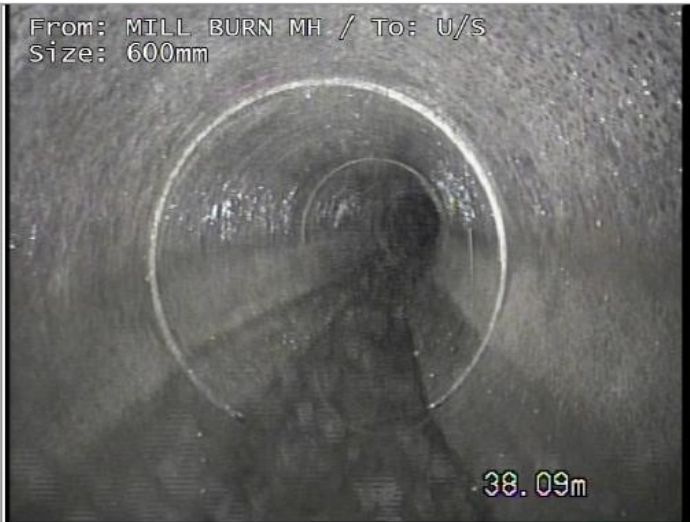
Junction at 10 o'clock, diameter 150mm
