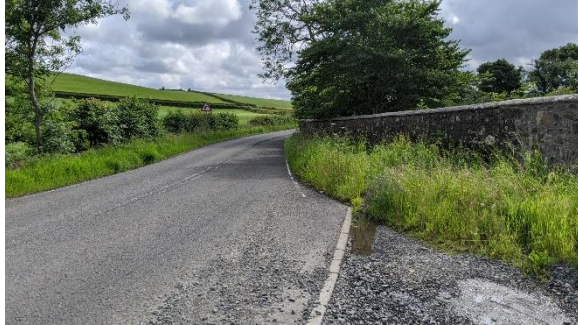
View at site entrance looking south along road edge
