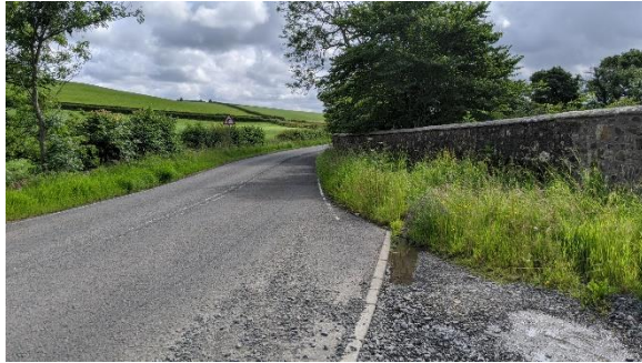
View at site entrance looking south along road edge
