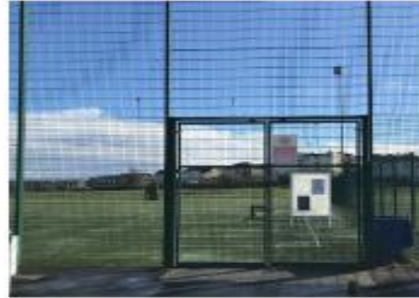
EXISTING GATE 1 (3.18m HIGH x 2.95m WIDE)
