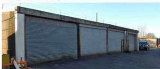
Existing Equipment Storage Building
