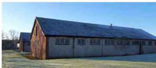
Existing Pavillion Building
