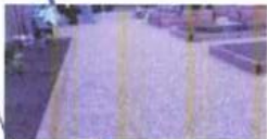
2mtr/1mtr wide Wheelchair Friendly Self Binding Gravel Paths
