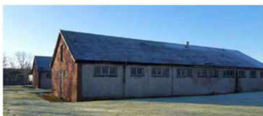
Existing Pavillion Building
