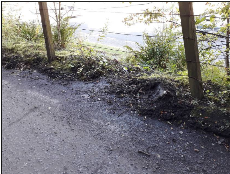
Plate 16– Pathway cut into northern side of Marypark Road to assist drainage down the embankment.
