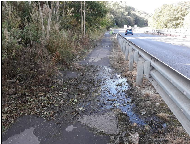
Plate 14 – Seepage from embankment onto footpath adjacent to A8.
