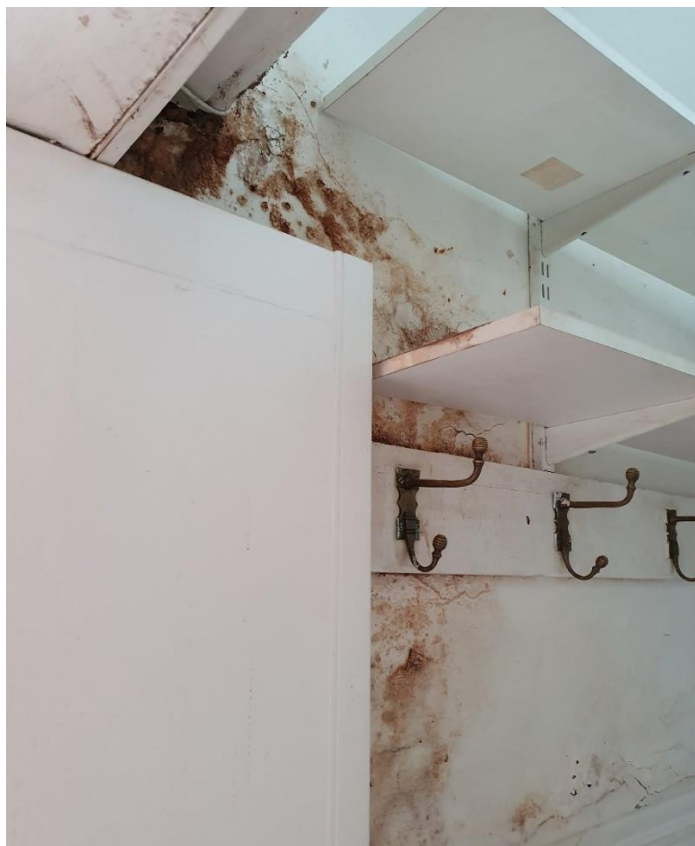
Figure 4 – Interior of West Lodge, showing damp and water ingress
