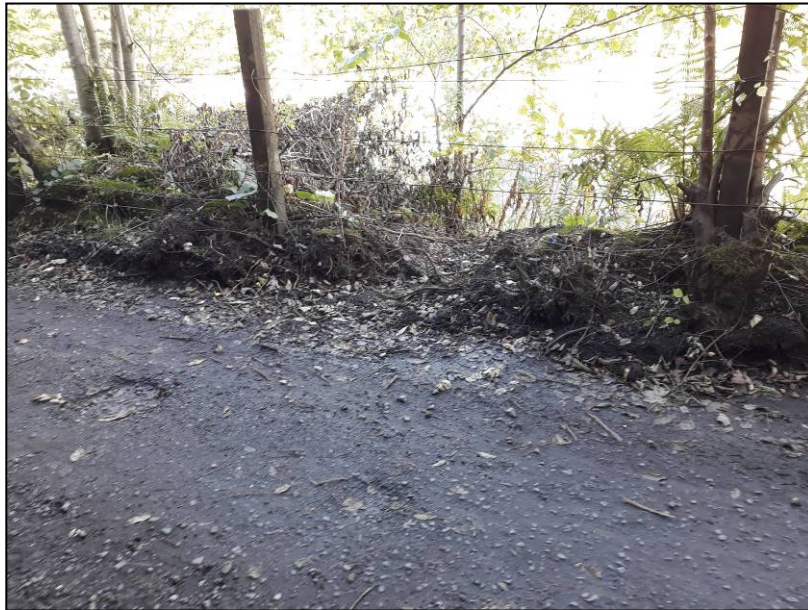
Plate 17– Pathway cut into northern side of Marypark Road to assist drainage down the embankment.
